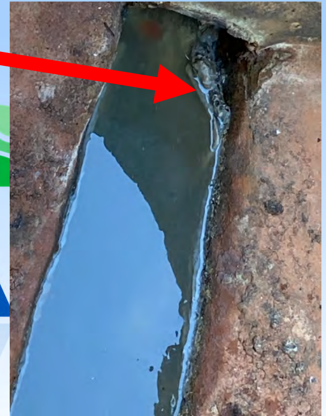
Grease build up on an OJRSA line that was "jetted" from a Member City line into the trunk sewer (October 2023)
