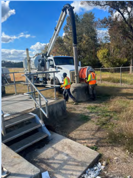
Cleaning grit and debris from 36-inch sewer along Coneross Creek
