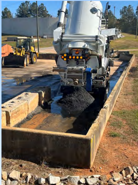
Cleaning grit and debris from 36-inch sewer along Coneross Creek
